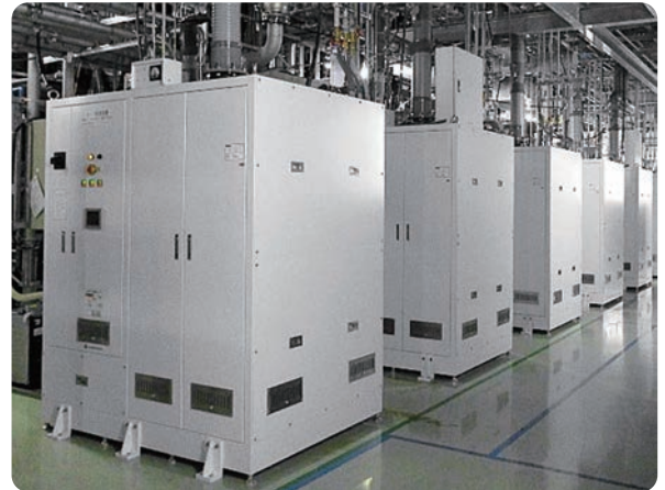
PFC Abatement Equipment
