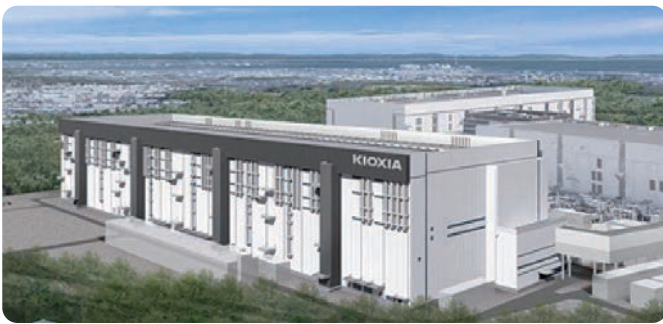
Image of the completed Fab7
