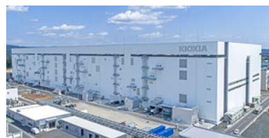
Kitakami Plant (Kioxia Iwate Corporation)
