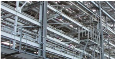
Overhead piping (no buried piping) Reduces the risk of soil contamination
