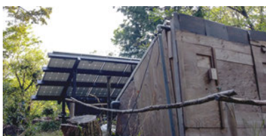
Solar battery panels powering the on-site equipment
