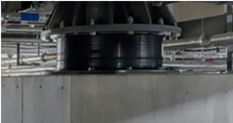
Plant seismic isolation device
